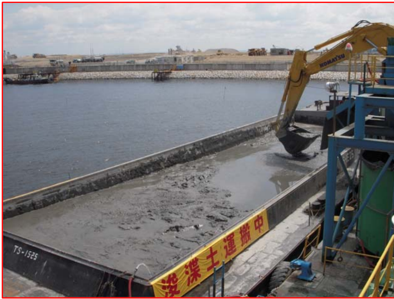
Dredged soils at Haneda airport construction
