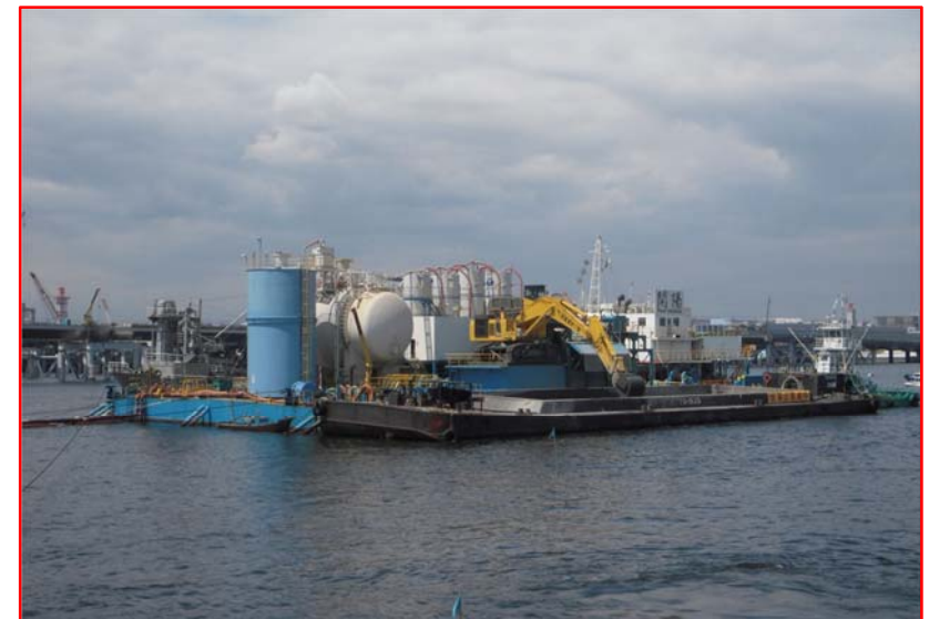
Special working ship for cement treatment at Haneda airport construction
