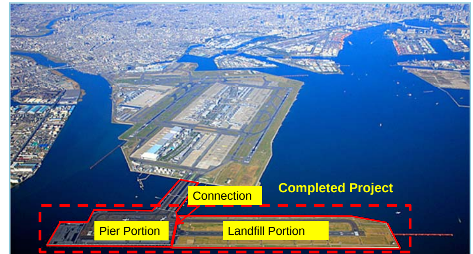
New runway at Haneda Airport (D-runway)
