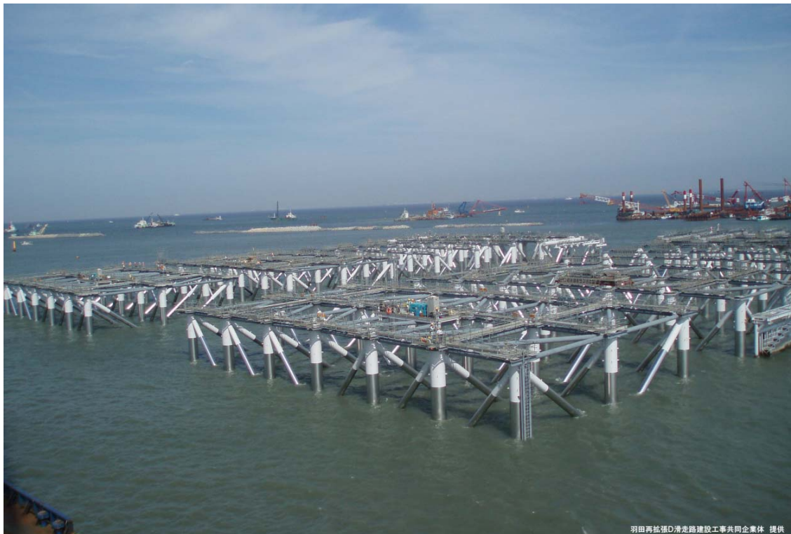
Fig. 1 Jacket structure of the D-runway of Haneda airport (connection bridge) ( http://www.pa.ktr.mlit.go.jp/haneda/haneda/haneda_saikaku/photo/b/080625b.jpg )
